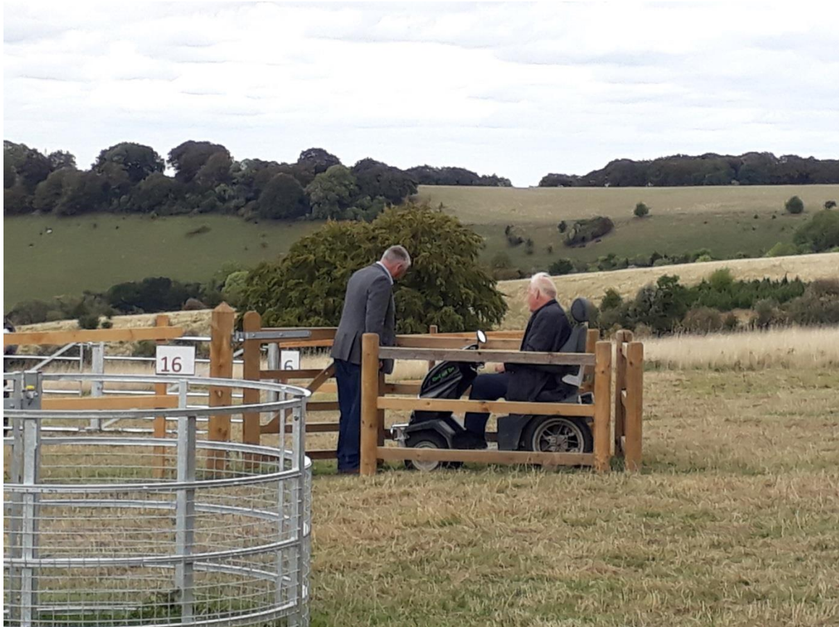
A timber kissing gate with bypass. Although to British Standard, you can see that this only just fits the mobility scooter. In the foreground is a metal kissing gate with 'radar' key opening bypass.
