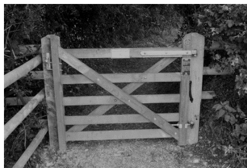
The original footpath stile replaced with a gate and new surfacing
